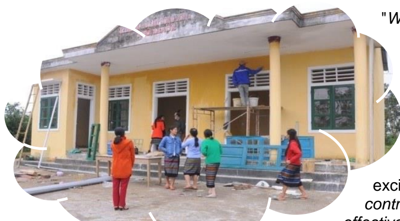
Community members are monitoring the culture house upgrade
